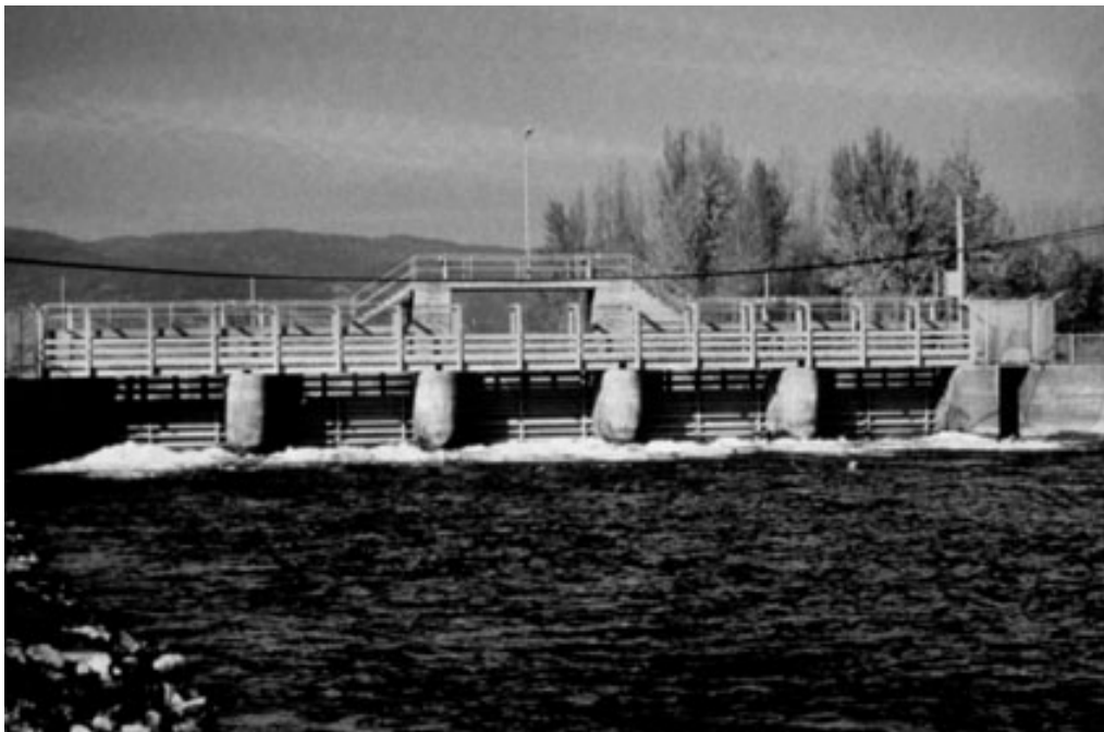
Figure 20. The same site pictured in Figure 18, as seen in 1983. The lake and river levels are now controlled by a dam and the river has been straightened, channeled and bordered by dykes. (Photo: Robert A. Cannings).
